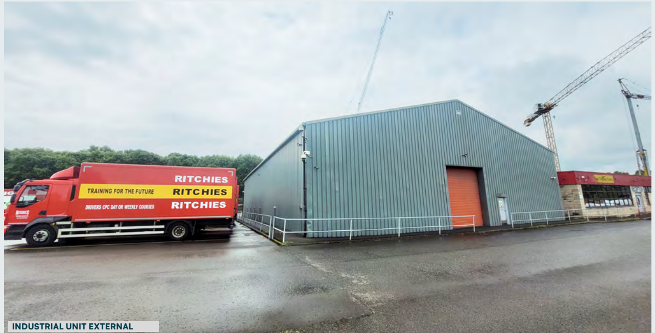
INDUSTRIAL UNIT EXTERNAL
